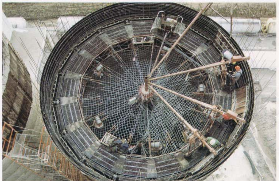
WOODSTOCK JOB using MWI's jumpform system involved smaller crew than slipform operation. Instead of using expensive, long-reach cranes to bring up materials, lifting was done by self-climbing form system.
