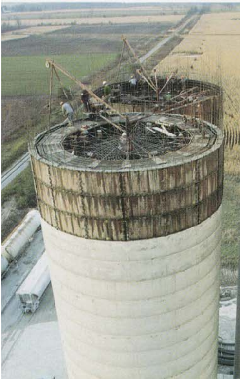
WOODSTOCK JOB using MWI's jumpform system involved smaller crew than slipform operation. Instead of using expensive, long-reach cranes to bring up materials, lifting was done by self-climbing form system.
