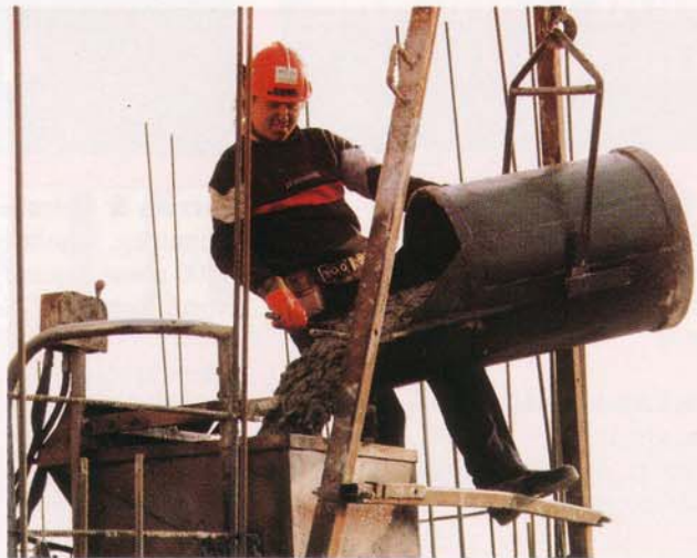
JUMPFORMING time spanned 11 weeks, with both silos climbing at once.
